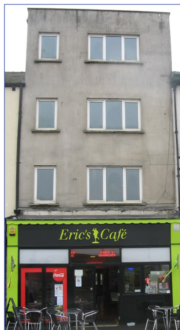
245 Marine Road Central (above, before and in progress)
