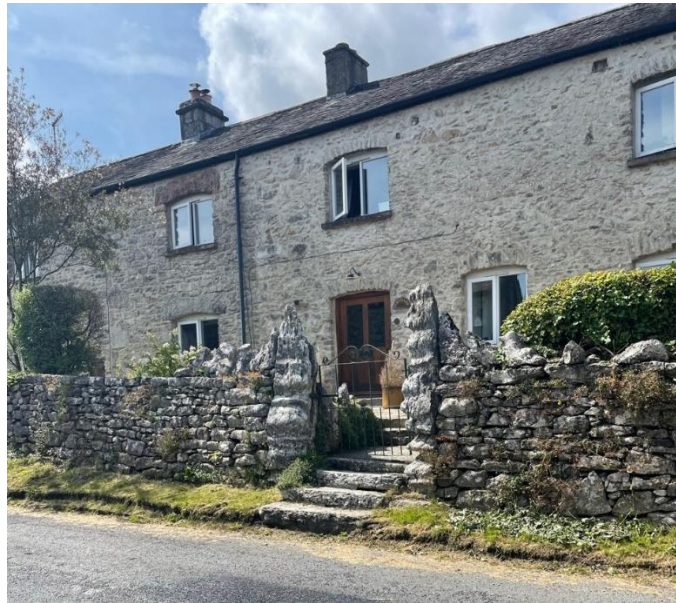
Figure 55: Boundary wall to Fernbank, 27 Silverdale Road
