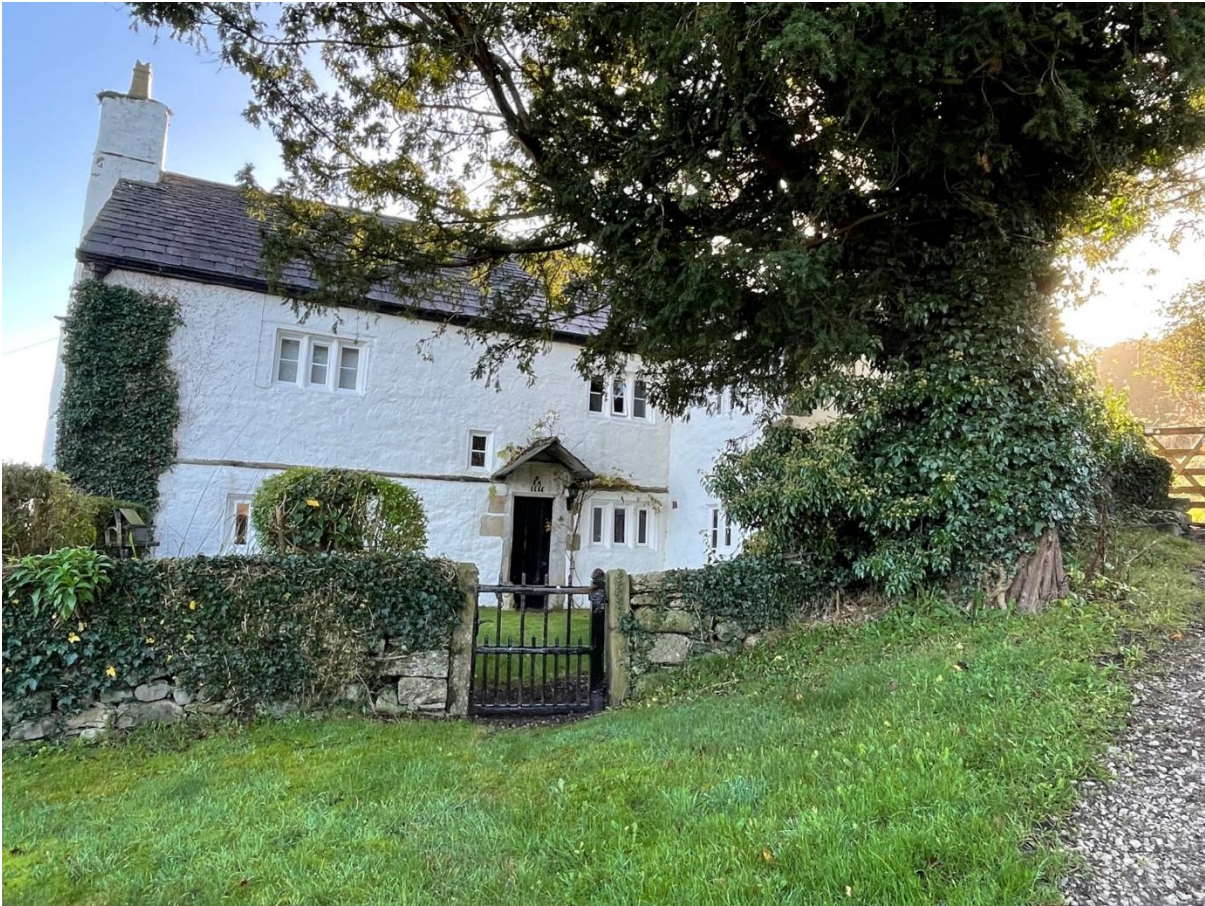
Figure 38: Storrs Farmhouse (grade II), with a 1666 dated lintel stone.
