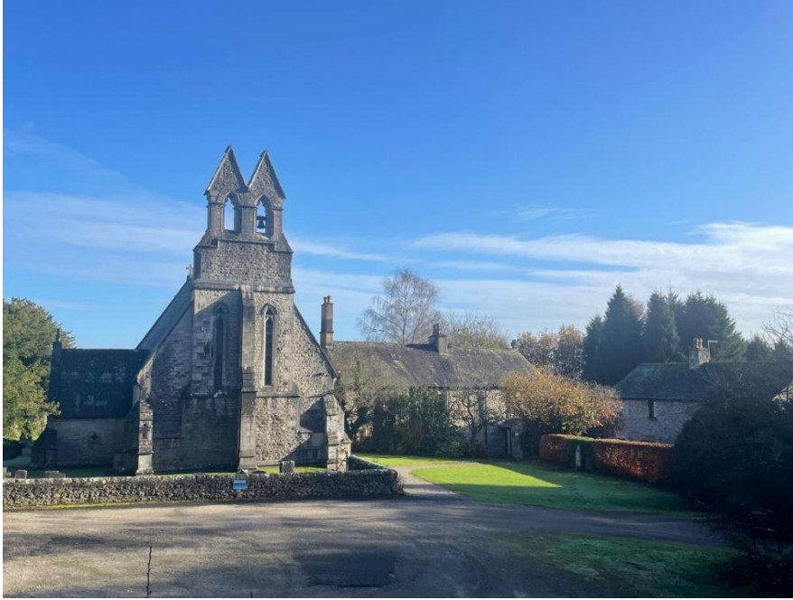
Figure 71: View of St Mary's as Yealand Conyers is approached from the south
