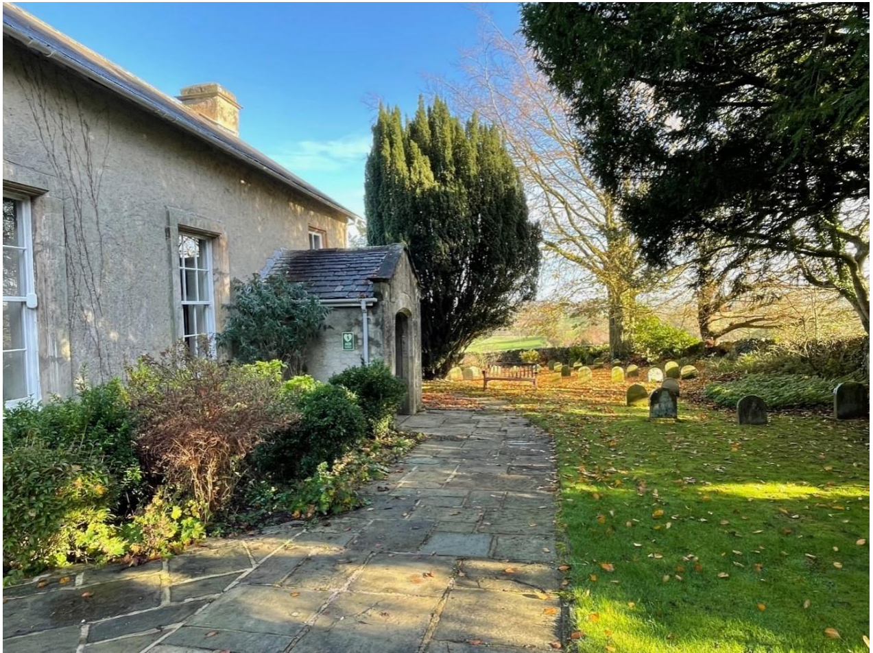
Figure 28: Yealand Quaker Meeting House (grade II*), 1692
