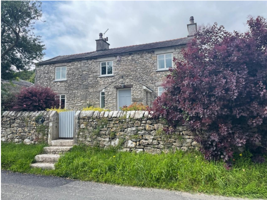
Figure 77: Greenthorne Farm, 35 Silverdale Road, positive unlisted building (and NDHA)
