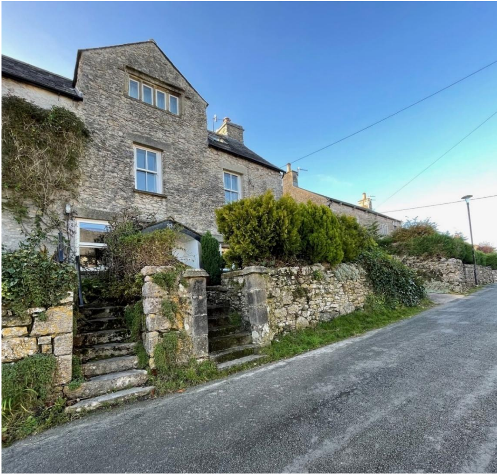
Figure 36: C17 Yew Tree House (grade II), with a stone gabled attic dormer and distinctive four-light mullioned window.
