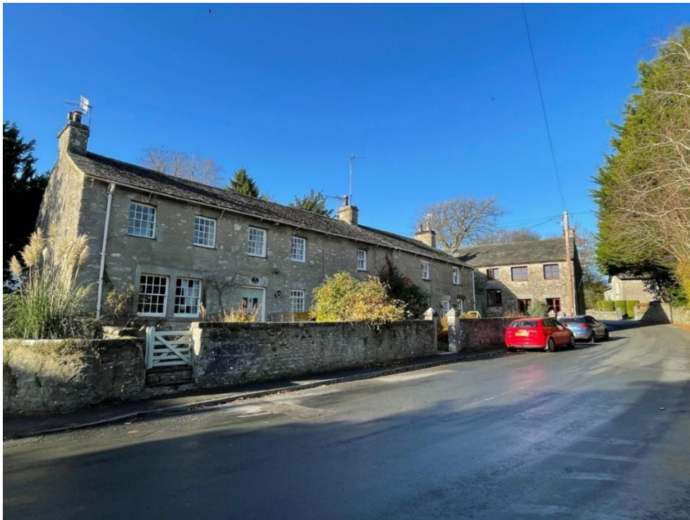
Figure 24: No.s 5-9 Yealand Road (grade II) and the Coach House, handloom weavers' cottages and flax dressing mill dating from the early C19
