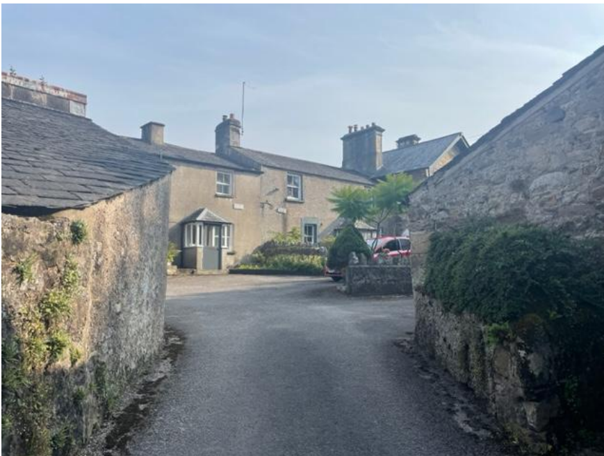
Figure 45: Close at rear of Green Leigh and Plough House. Forecourt includes surviving cobbled surface
