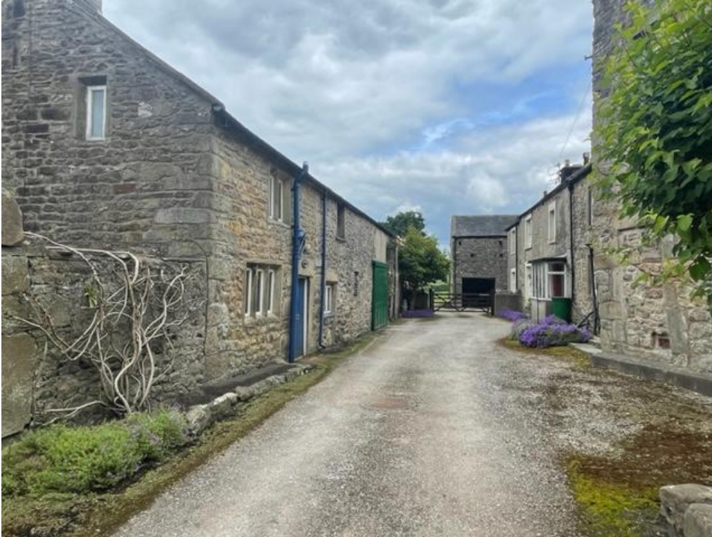
Figure 44: Close to rear of Hogarth House
