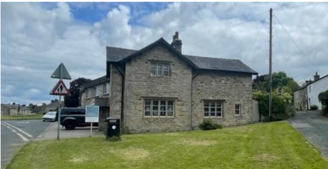
Figure 27, The Gables, a mid-C19 house
