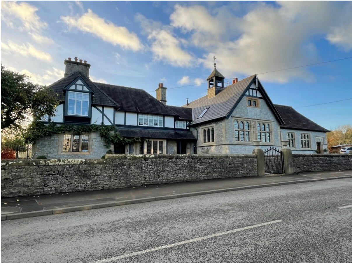
Figure 16: Paley & Austin's School & School House, 1875 (grade II listed)
