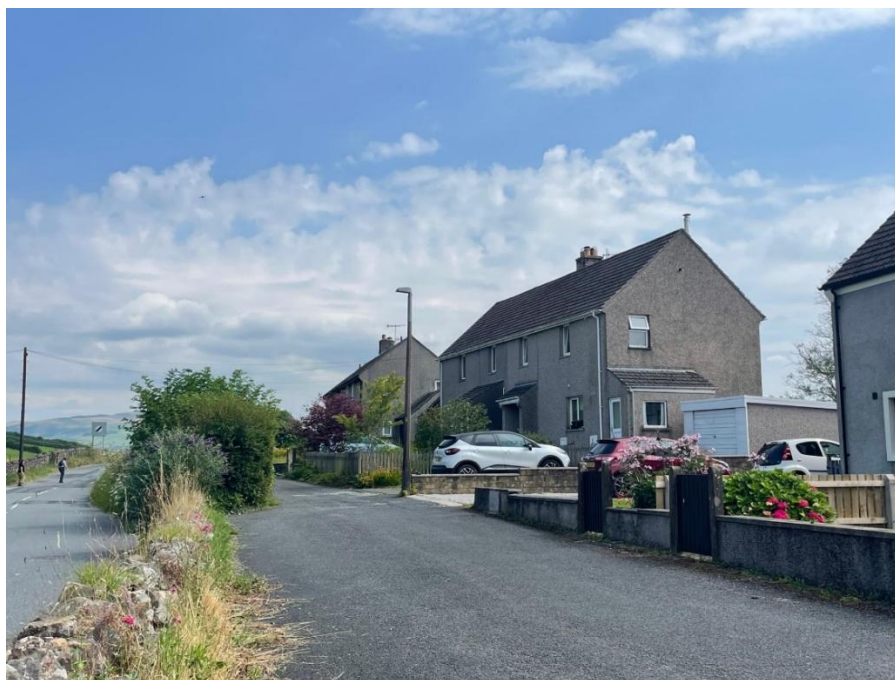
Figure 44: Mid-C20 Crosslands development to the north east of the conservation area
