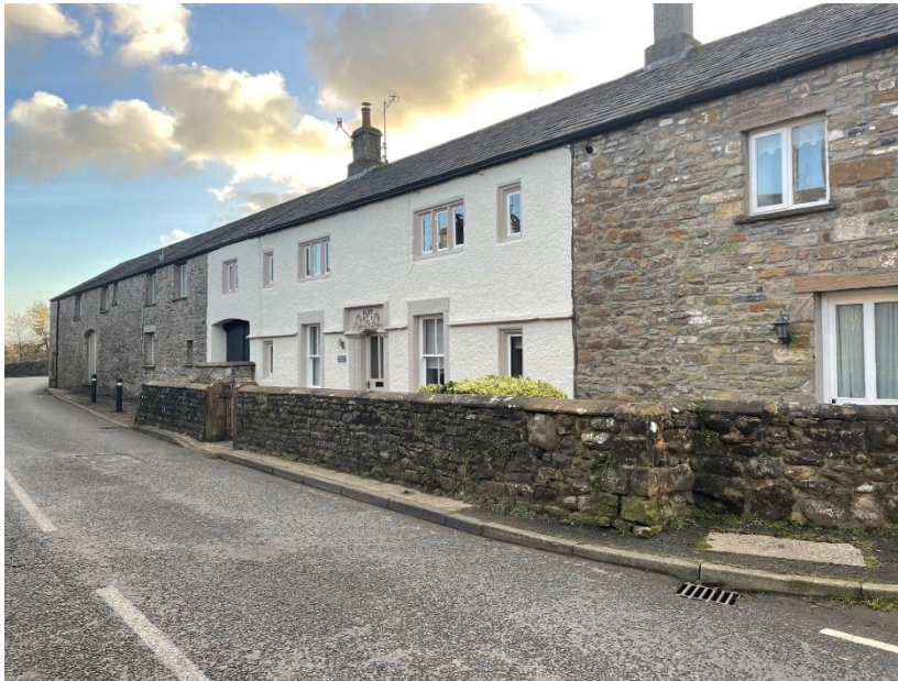
Figure 15: Malt Kiln House, 1687 (grade II listed)
