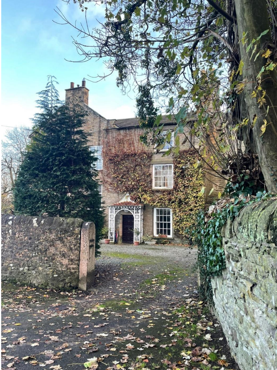
Figure 30: The Old Rectory, 1728 (grade II), slobbered north elevation to Church Street
