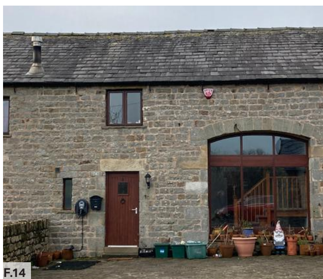
Figure 14: Converted barn with traditional stone elevations and slate roof
