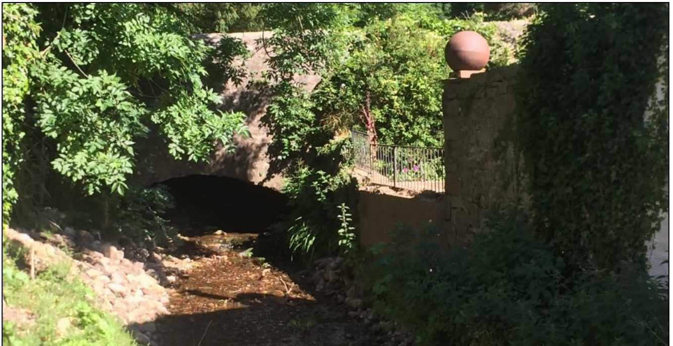
Figure B-4: Looking upstream at Church Bridge.
