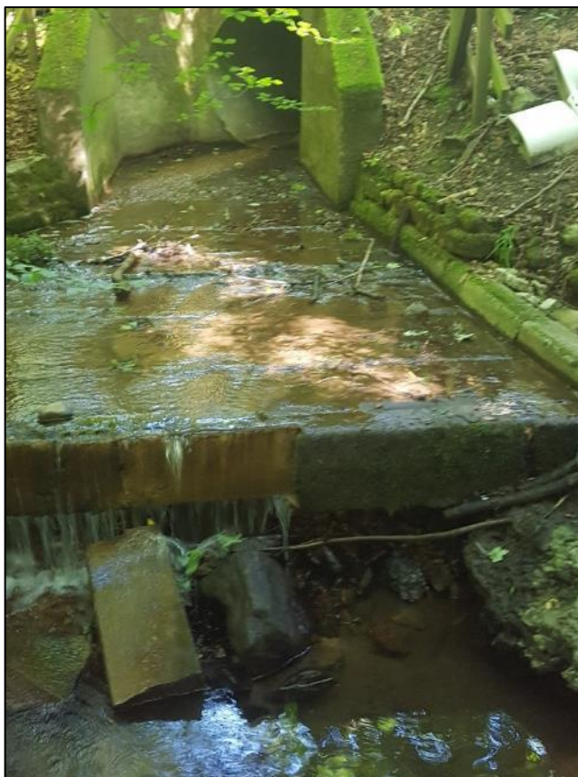
Figure D-7: Looking upstream at the outlet of Graveyard Culvert
