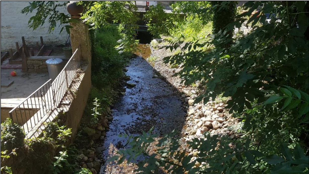
Figure B-2: Looking downstream at White Lion Bridge
