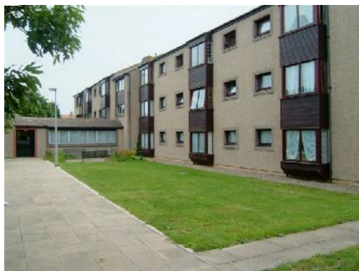
Council owned housing at Kingsway Court, Heysham
