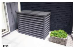
Figure 53: Air source heat pump housing covers the unit and harmonises with the building aesthetic
