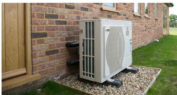
Figure 51: Air source heat pump unit
