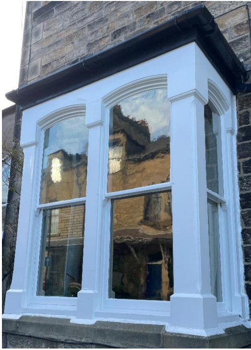
Figure 9: Characterful historic glazing in an 1870s house. This is likely to be drawn sheet glass.
