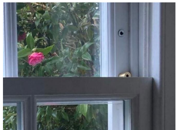
Figure 13: Brass restrictor. This can be unscrewed and moved into the alternative position with a key.
