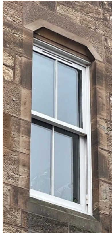
Figure 5: Timber sash window with surface mounted trickle vent
