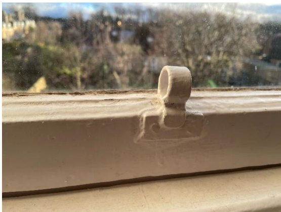
Figure 11: an over-painted brass sash ring lift
