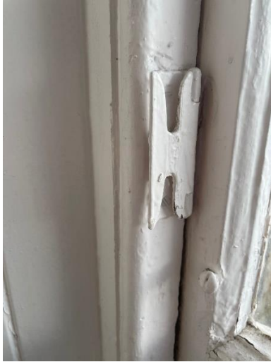
Figure 14: A Simplex hinge, with the locating screw fixed into the bottom sash, brass over painted
