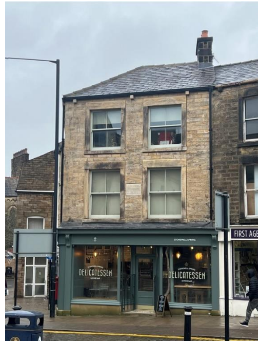
Figure 4: Replacement Accoya double glazed sash windows at Stonewell, Lancaster. Due to its location at a busy junction, a higher acoustic performance was required, necessitating the use of plant-on glazing bars.
