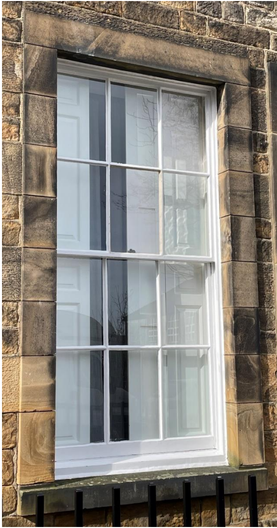
Figure 1: A sash window with operational internal shutters. Shutters greatly help a window's thermal performance.
