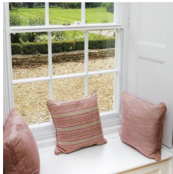
Figure 2: Vertical sliding sash secondary glazing system which enables the shutters to remain operational (credit: Storm Windows Limited, https://www.stormwindows.co.uk/ )
