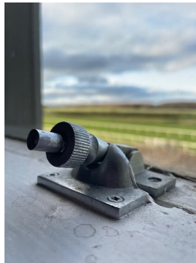
Figure 6: A Brighton fastener which can be unscrewed or tightened to control the ventilation, as well as for security and safety purposes
