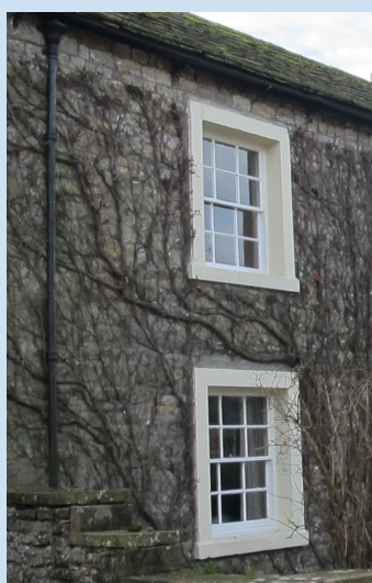
Fig. 30 Caulking House retains the traditional 6-over-6 sash window fenestration.
