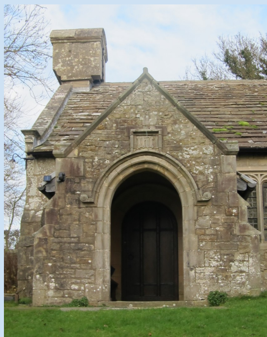
Fig. 4 St John Baptist church is grade II*. The building has parts which date back to the 15th century. A lot of the church was restored by local architects Austin and Paley in the late 19th century.
