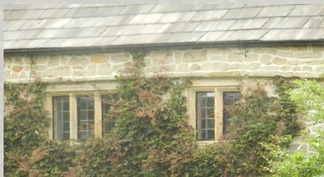
Fig. 20 Mullioned windows have been well retained at Pool House and contribute to the historic legibility of the building.
