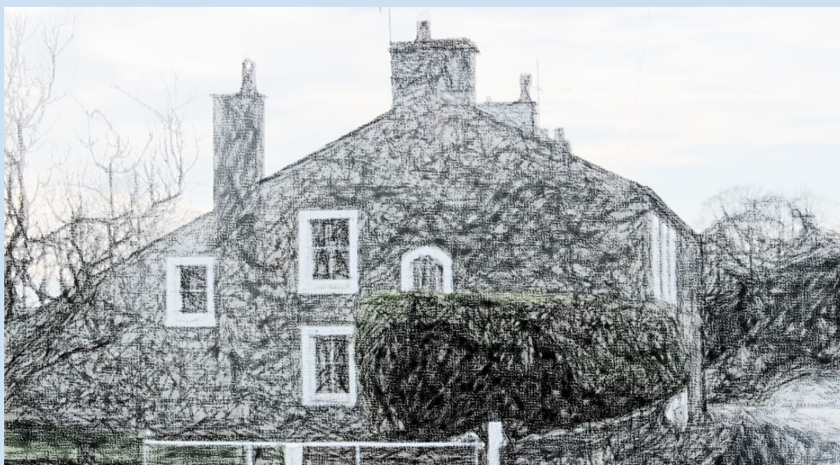
Fig. 2 Sketch of Chapel Cottages in Arkholme with a catslide roof on the outshut. The cottages have retained their architectural detailing, such as sash windows.
