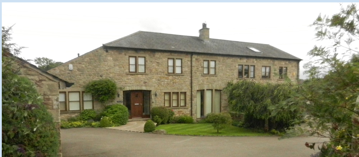
Fig. 5 Goss Lodge appears on the 1845 OS map as part of the land of Goss House. It has been converted to residential use, but like many other buildings in Arkholme it has retained its traditional barn door openings.
