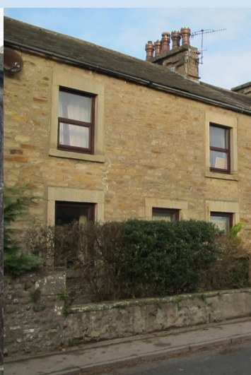
Fig. 31 Some traditional sliding sash windows have been replaced with unsympathetic modern mock-sash casement opening windows.
