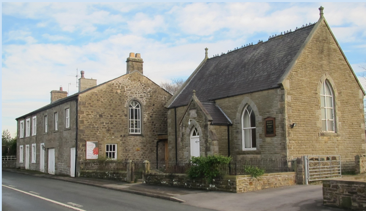
Fig. 28 The Methodist Church (on the right) shows Gothic-revival detailing in the pointed arched windows and doors. The Chapel Cottages (on the left) are constructed more traditionally with an arched window on the gable end.
