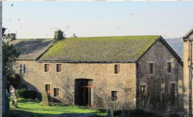
Fig. 18 This mid-18th century barn is attached to Church Gates Cottage and has been converted to residential use.
