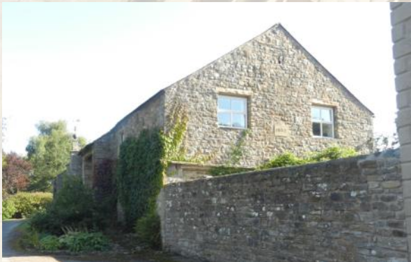
Fig. 17 Late-18th century detached barn, which has been converted to residential use.
