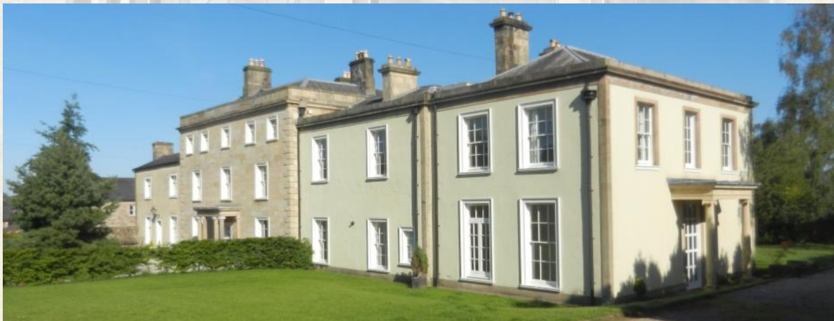
Fig. 19 Melling Hall is a mid-18th century house which demonstrates the Georgian era's neo-classical architectural influence.
