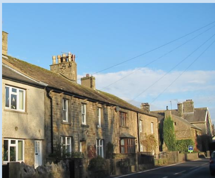
Fig. 29 Town End House (in the centre) has origins from late-17th century with a datestone reused on the rear extension of '1673'.
