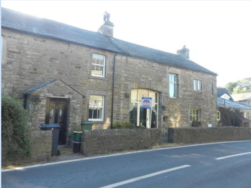
Fig. 8 Ash Lea and The Old Forge are traditionally constructed in sandstone with slate roof. The Old Forge has retained architectural detailing of its previous agricultural use as a barn with the segmental arched opening.
