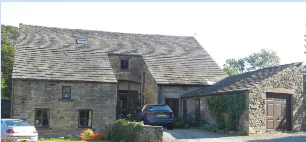
Fig. 14 Underhill is a late-18th century barn constructed in sandstone with a stone slab roof. In the late 20th century it was converted to residential use.
