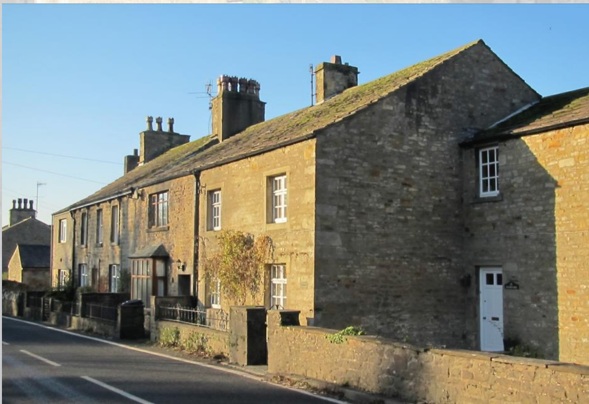
Fig. 6 View along the A683 of traditionally constructed terrace of houses, which have also retained traditional stone boundary walls.
