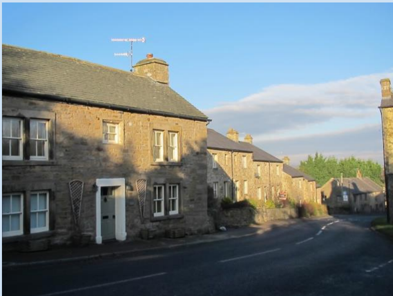
Fig. 9 Crow Trees farmhouse in the foreground is a 17th century farmhouse constructed in sandstone rubble and grey slate roof. Melling Brow in the background is modern terraced housing development which positively responds to the vernacular expression of Melling's conservation area.
