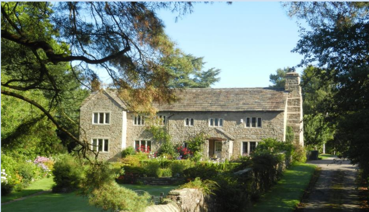
Fig. 24 Old Crowtrees dates from late 17th century, constructed in rubble sandstone with a stone slab roof to the front with a large projecting chimney stack to the right. To the left a gable projecting extension was constructed in a sympathetic style in the late-20th century.
