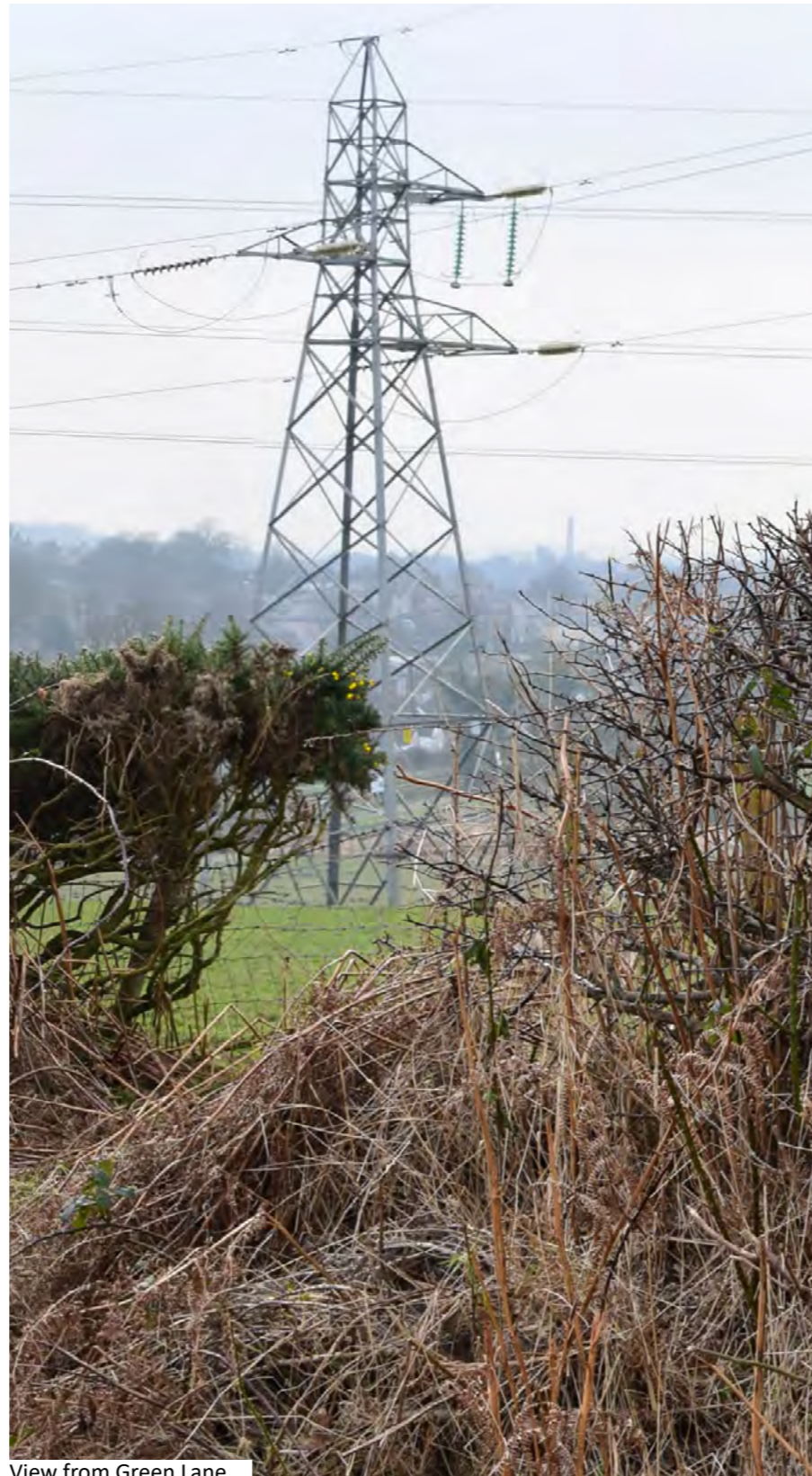
View from Green Lane
