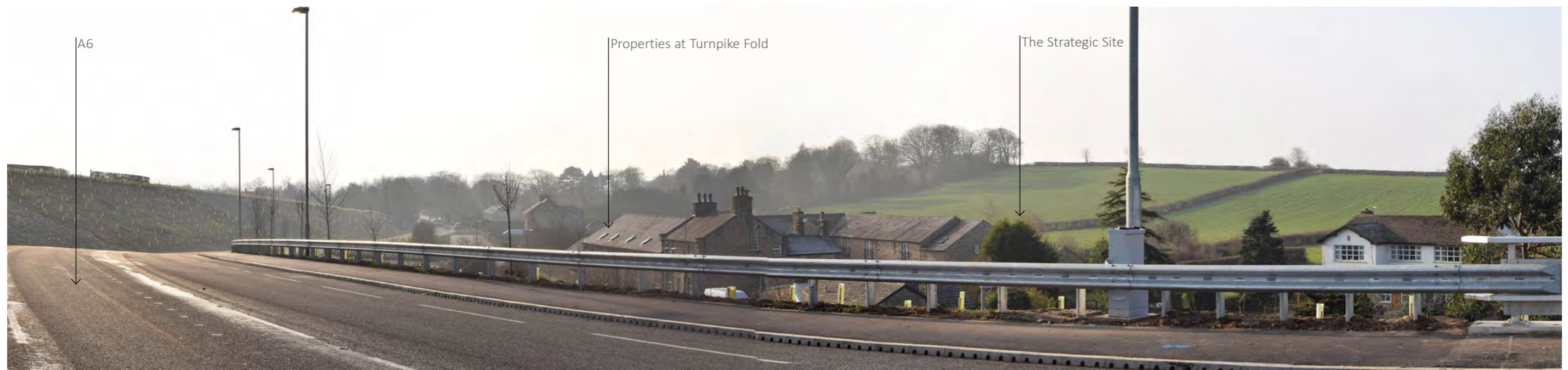
View from the A6 looking south and south west towards the Strategic Site
