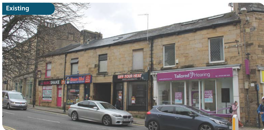
Existing view looking at the shops along the Stonewell Nose.
