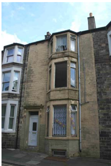
Inappropriate windows and door
