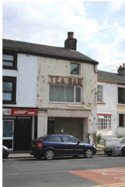
Vacant and in need of repair/restoration
