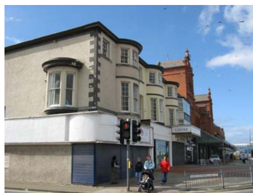
The bowed windows of Craven Terrace
