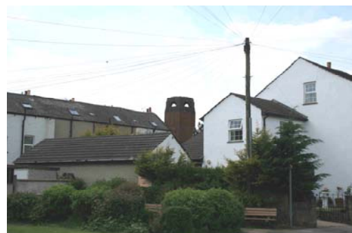
Fire Station tower
