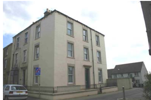
A stuccoed building with ashlar lines scored
