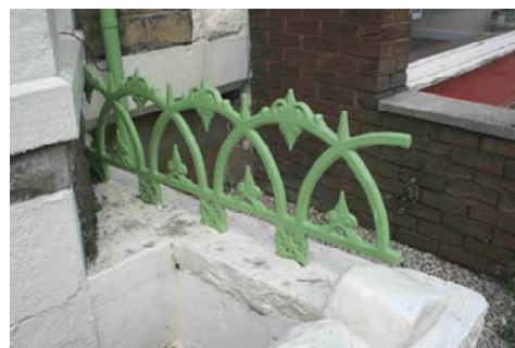
Remnants of the historic railing pattern
