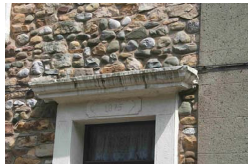
Cornice over door detail
