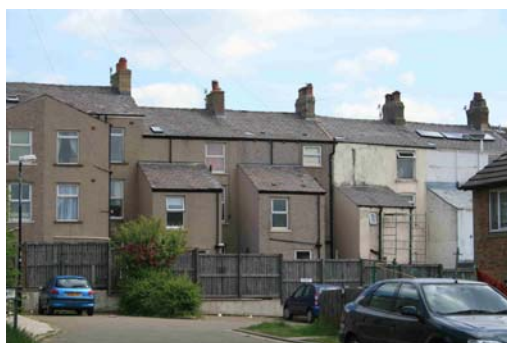
Two and three-storey outriggers
