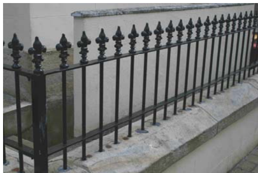
Newly reinstated railings
