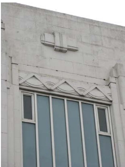
Woolworths Building detail
