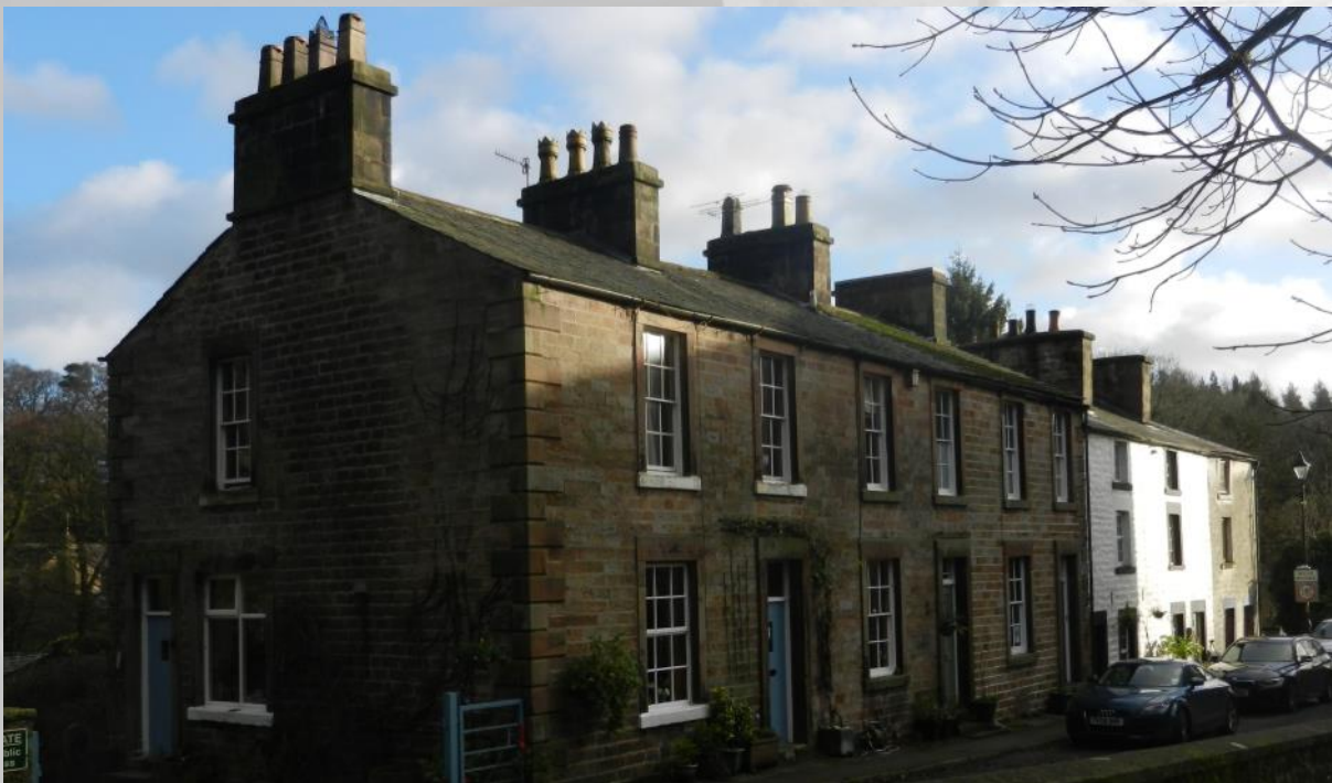
Fig. 28 Wagon Road terraced housing early 19th century - constructed in traditional materials such as sandstone, render and slate.
