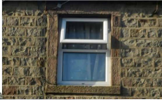
Fig. 27 Replacement of traditional timber sliding sash windows with PVCu alternatives.
