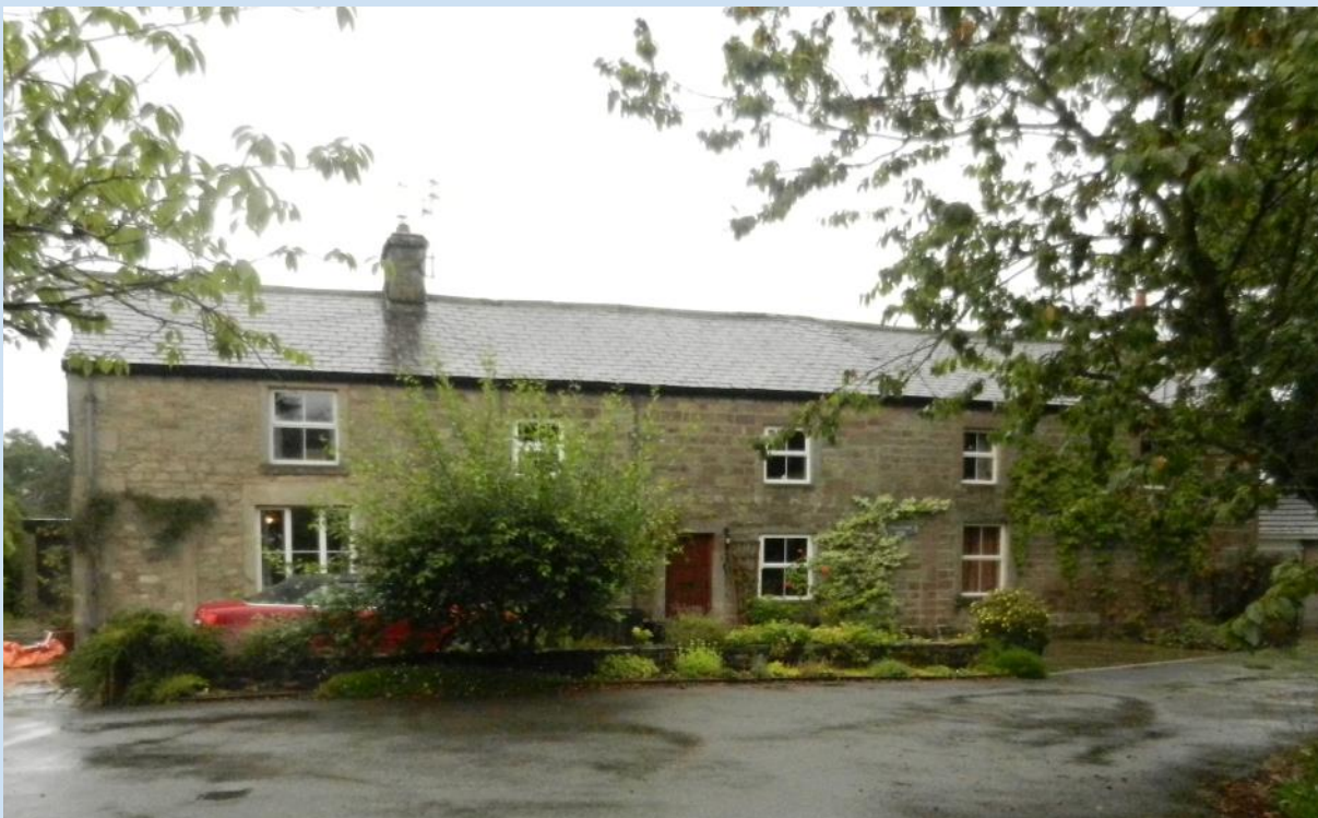
Fig. 33 Common Bank House constructed in random coursed sandstone and grey slate roof. Originally the property may have been a long house but has been largely extended and altered with the addition of windows, doors and chimneys.
