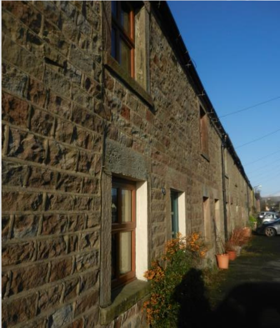
Fig. 24 Sandstone walling predominantly characterises the historic buildings in Upper Dolphinholme, some are also traditionally rendered along Wagon Road.
