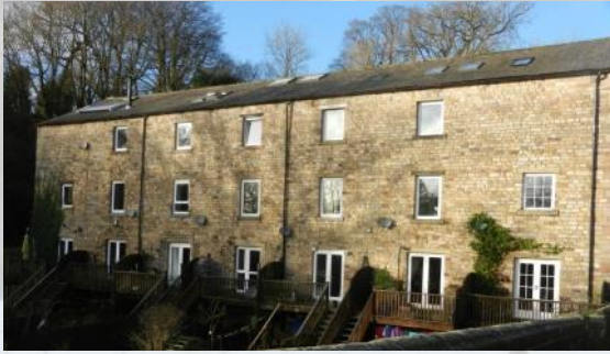
Fig. 17 The 19th century warehouse was converted to housing in late-20th century.
