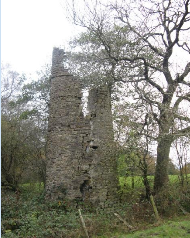
Fig. 14 The chimney stack was built in the early-19th century to improve efficiency of the fire and draught in the mill.
