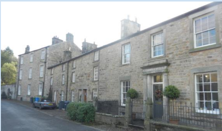
Fig. 12 Derham House in the foreground has a porch with Doric columns and traditional six-over-six paned sliding sash windows. The house is enclosed by a low stone boundary wall with railings.
