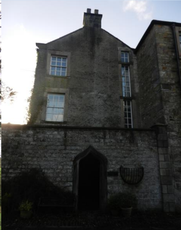
Fig. 15 Old Mill House, dates from 1800. The boundary wall also dates from 1800, with an ogee headed doorway,
