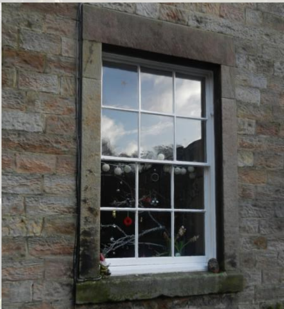
Fig. 25 Traditional early-19th century timber sliding sash window with slim glazing bars. Such features contribute positively to the historic architectural interest of the area.
