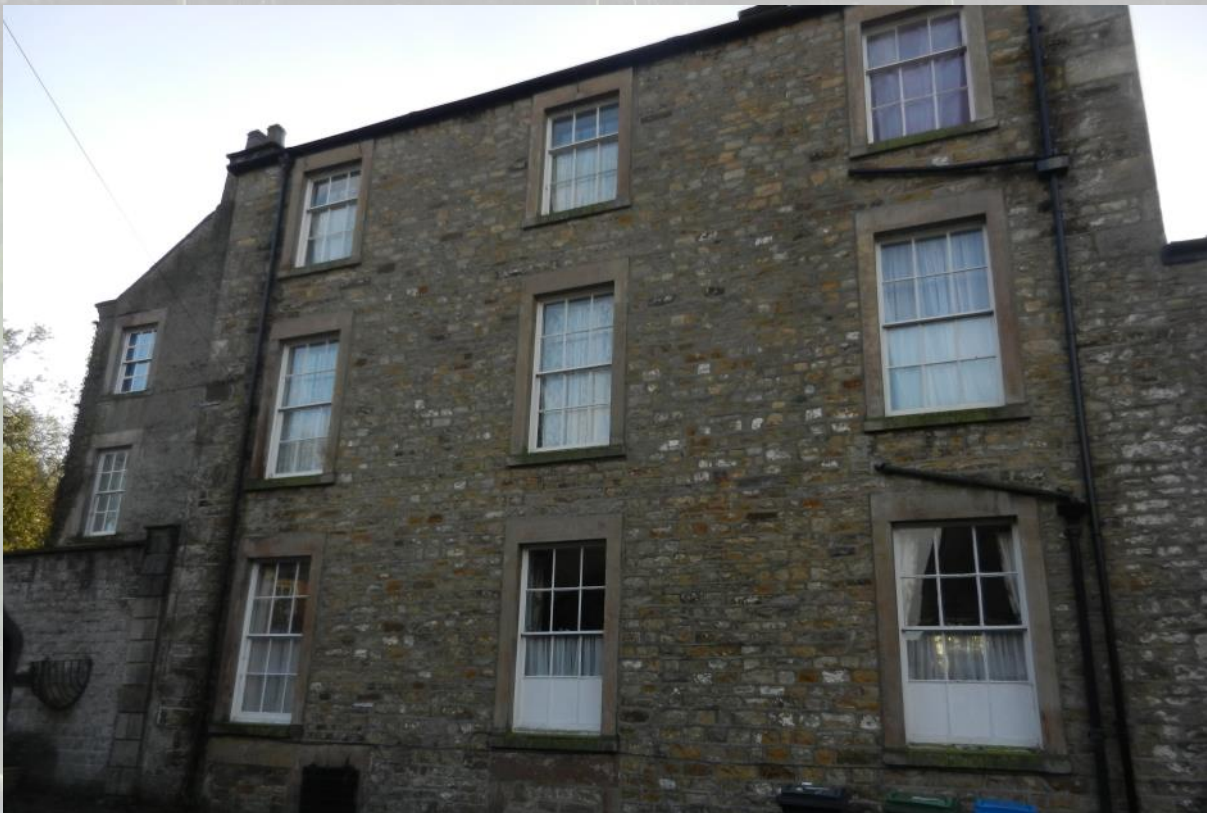
Fig. 11 Woodcock Hall dates from 1800, it is constructed in local sandstone rubble walling and grey slate roof. It shows influence of national architectural styles of the Georgian period as it is designed in a simple Georgian style with symmetrical façade.
