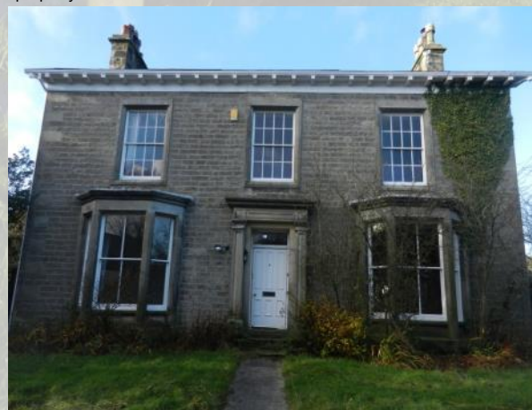
Fig. 8 St Mark's Vicarage was built in the late-19th century in Victorian eclectic style with Doric columns and two canted bay windows.
