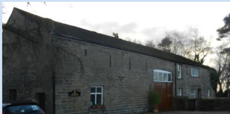
Fig. 32 Corless Farmhouse with attached barn traditionally constructed in sandstone. Agricultural details, such as breather holes and a segmental barn door opening, are still visible.
