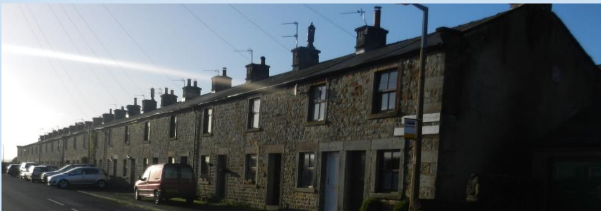
Fig. 16 1-18 Corless Cottages are two storey terraces constructed in coursed sandstone and grey slate roof. Each property has two windows, which originally would have been timber sliding sash, with stone surrounds. This terraced is located south east of 19-28 Corless Cottages, which are three storey grade II listed terraces.
