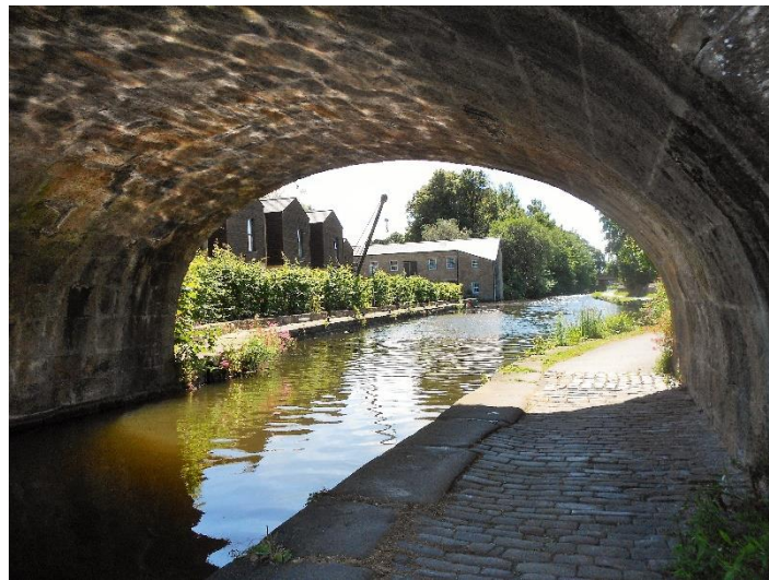
Canal Bridge adjacent to Aldcliffe Yard
